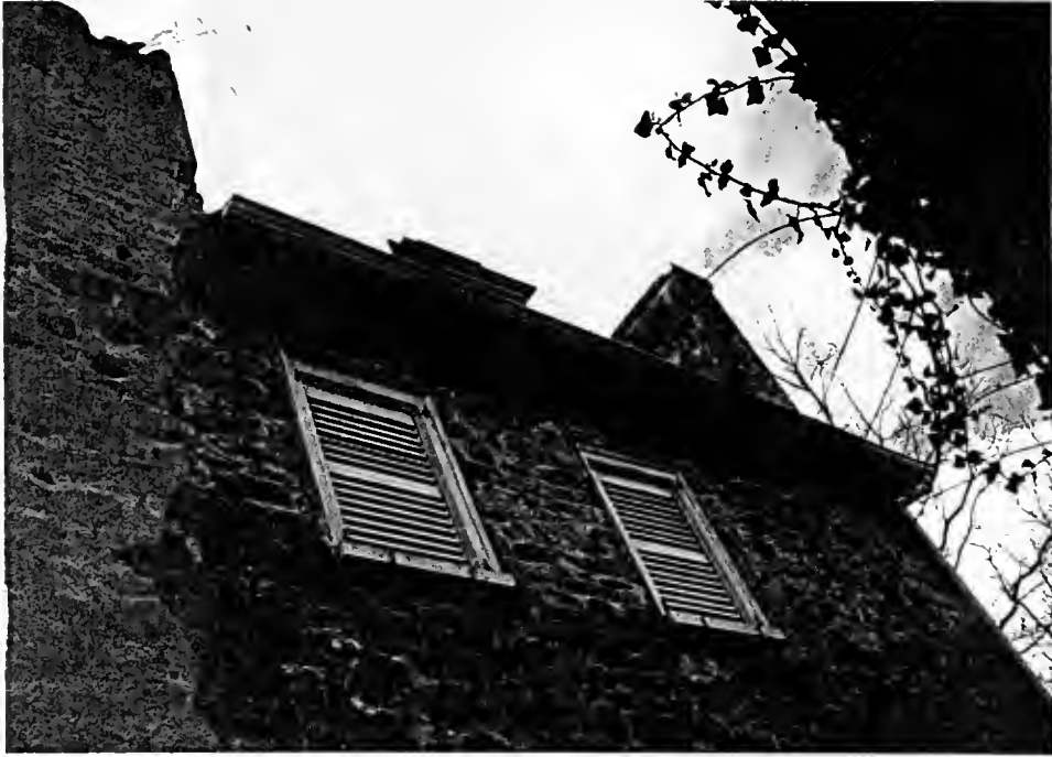
Figure 16: Exterior of the Pawling section, east elevation
